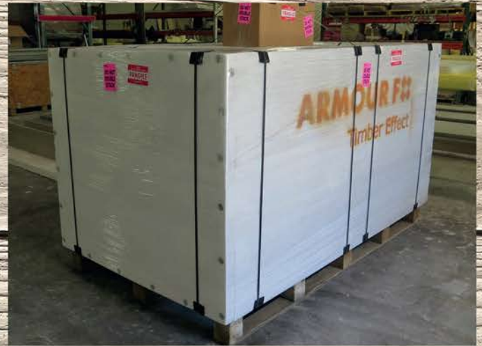
Panels shipped to site in custom made EPS crates.
